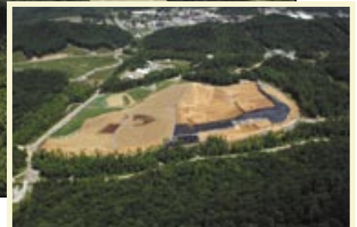
Solid Waste Storage Area 5
