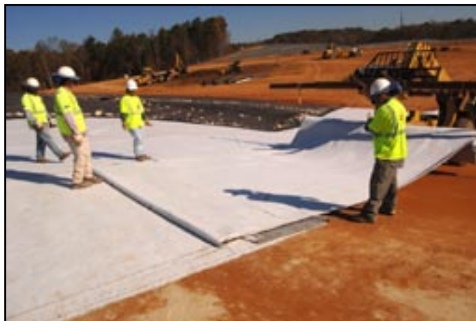
Liner placement over a Solid Waste Storage Area
